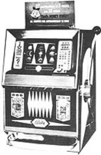
No one changed the basic design of Charlie Fey's three-reel slot machine for six decades. Outward designs changed, but even in the 1950s, the vast majority of slot machines were basically steel boxes containing three spinning reels based on Fey's original design.
